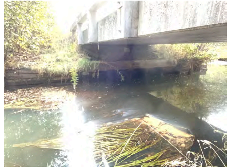
Right Bank Abutment when facing downstream
