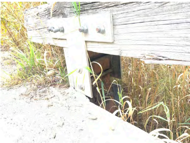
Rotten guardrails
