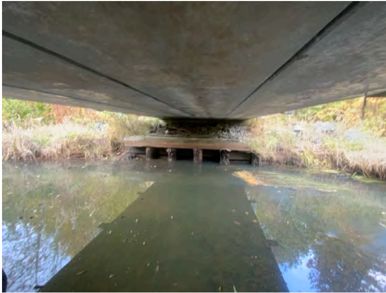
Left Bank Abutment when facing downstream
